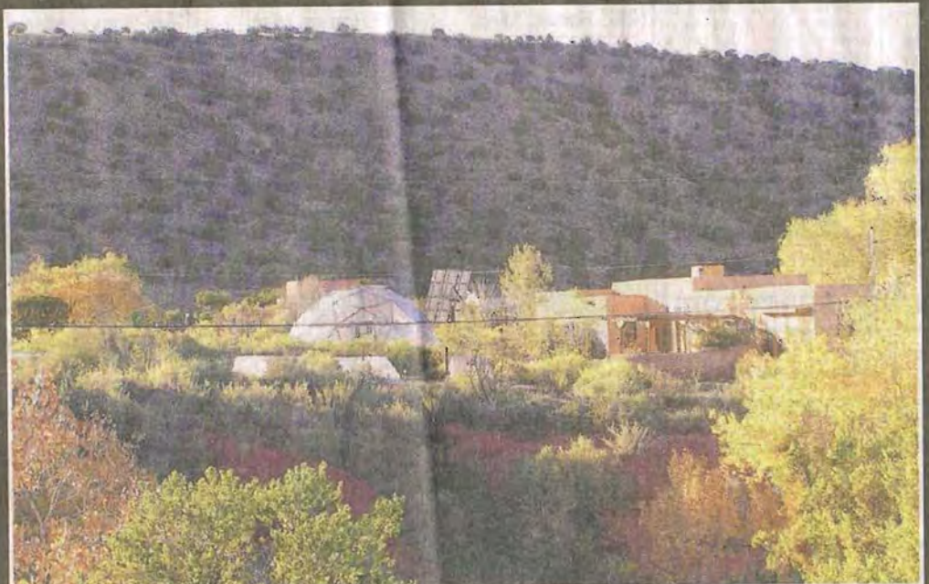
This home in Embudo is a work in progress. The nearly net-zero 3,000 square foot home provides some food for the occupants. Passive and active solar systems produce 95 percent of the heat and hot water. An interior atrium and attached greenhouse provide beauty, light and oxygen.
