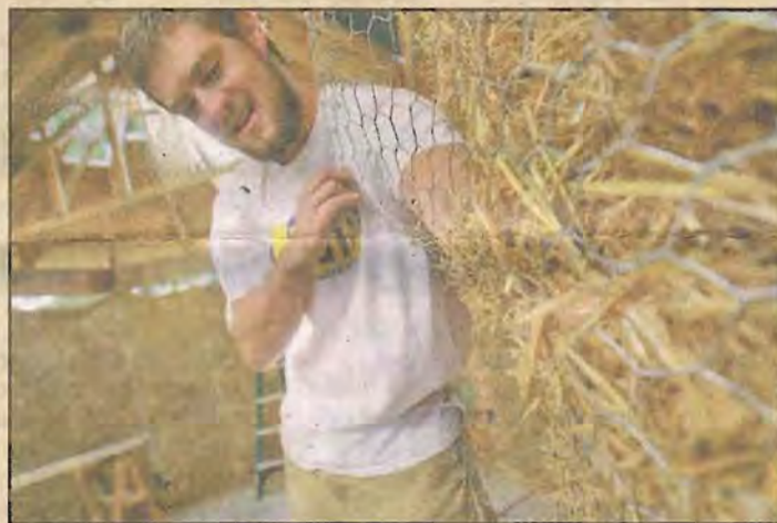
Above, Eric Basinger of Paja Construction Inc. stuffs straw behind metal mesh. The mesh eventually will hold the home's plaster or stucco. Below, Cadmon Whitty, owner of Paja Construction Inc., believes parts of straw-bale construction are doable by the homeowner/builder.
